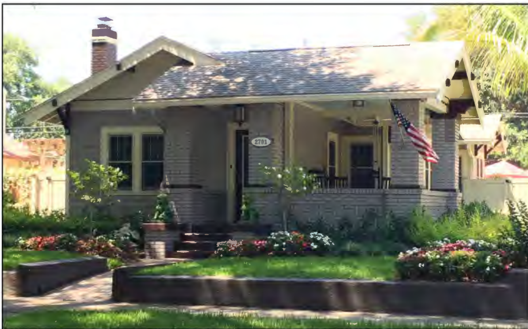
Figure 4: Bracket and beams that extend through decorative bargeboard at 2701 2 nd Ave N.
